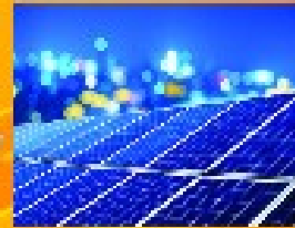
Solar Panel Campus
